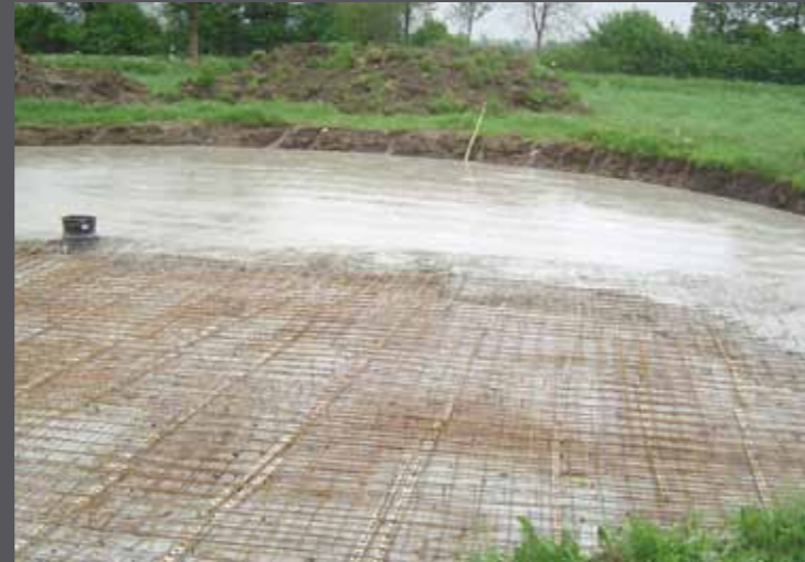
Base during concrete-laying
